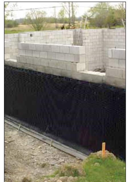
DMX AG™ applied to foundation wall eliminates the effects of Capillary Suction and Hydrostatic Load.
