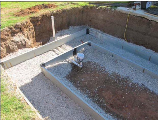
Figure 18: ICF pool foundation with gravel in place before installing rebar grid.
