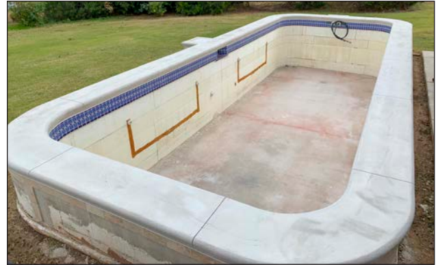
Figure 74: The pool coping is poured and forms stripped. Score with a concrete saw every 24"-36". Fill the seam with pool plaster, caulk, or another material.
