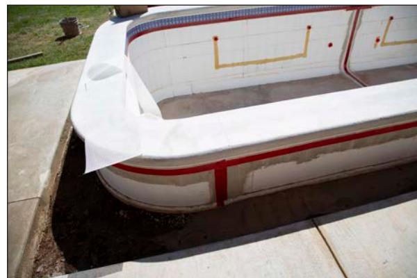
Figure 64: With the cove transition and pool cleaned for finish installation, stage mesh and other materials as needed.
