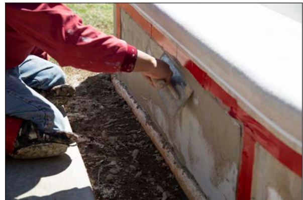
Figure 76: Additional BuildCrete material is used to embed the mesh completely and build up to the finished thickness.
