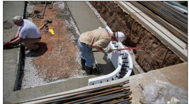
Figure 22: Pouring an ICF pool foundation and screeding the foundation level.
