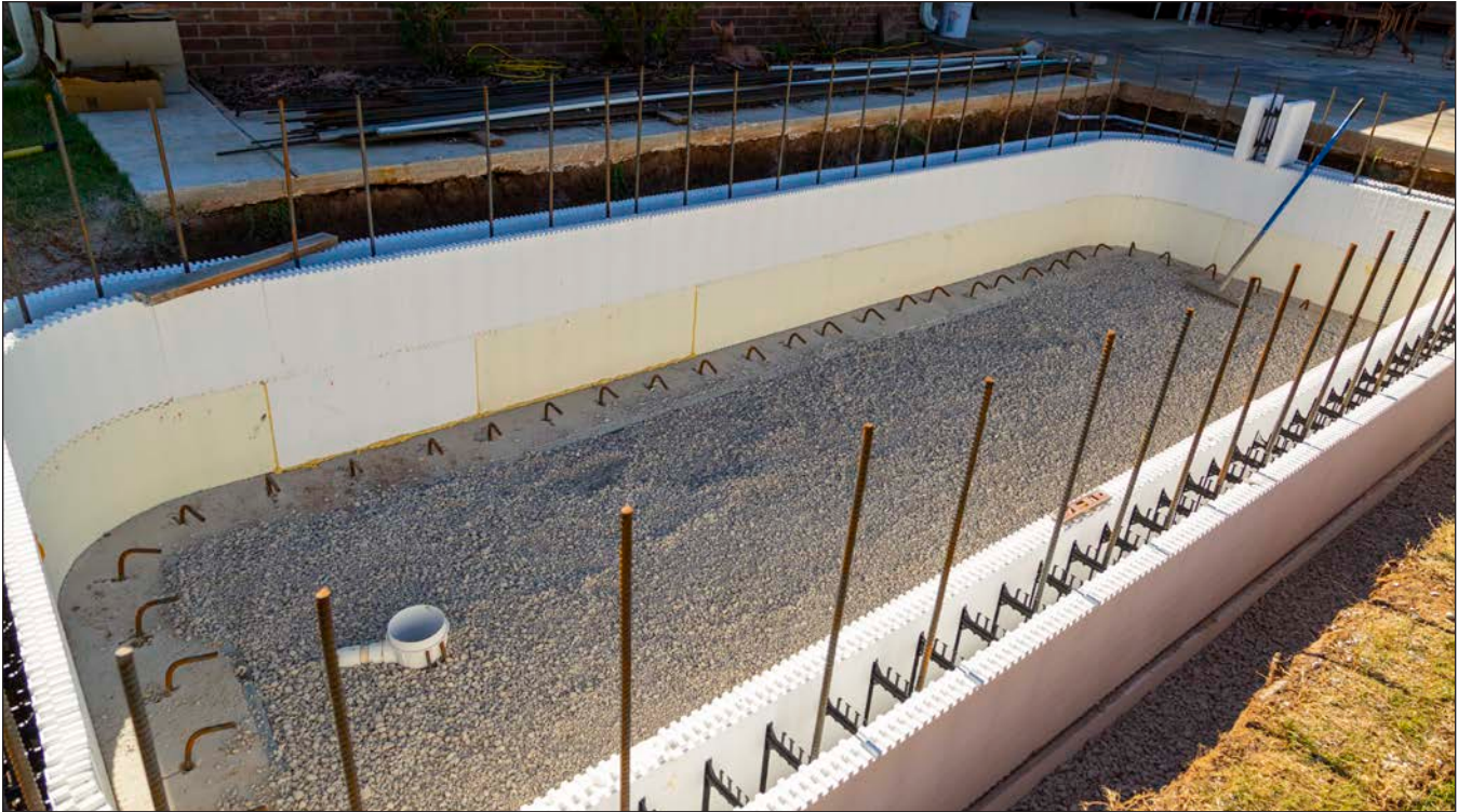
Figure 8: BuildBlock ICF Pool with footings poured and first two courses set.
