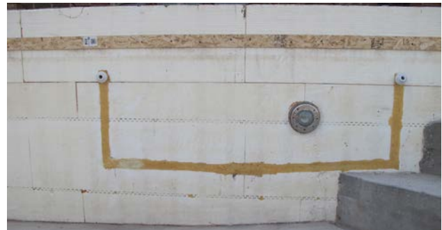
Figure 49: Pool return jets secured in place with foam adhesive and trimmed smooth for pool finish. Electrical light installed and ready for finish installation.
