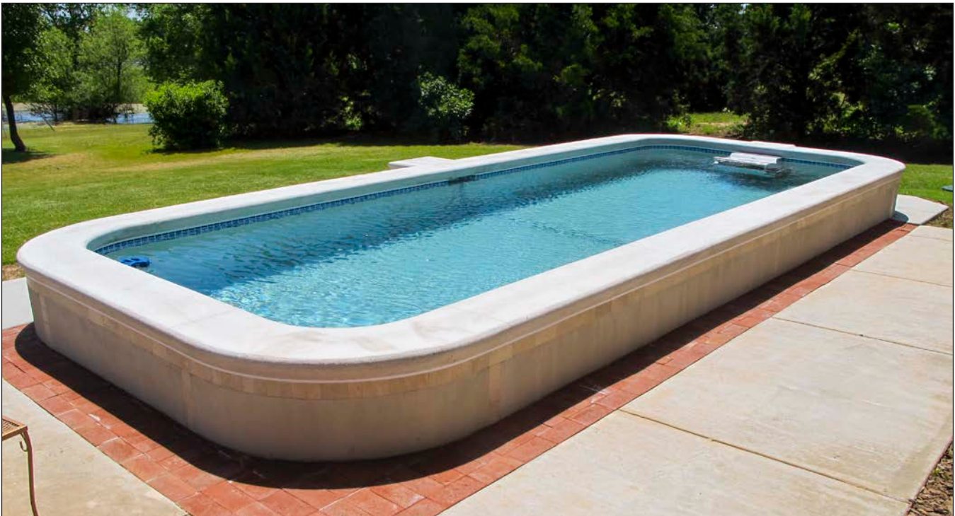
Figure 7: Completed BuildBlock Test Pool.
