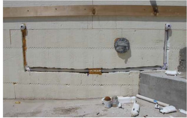
Figure 47: Pool return jets installed and connected to supply line via central coupler passing through sleeve in pool wall.
