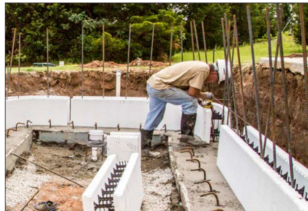
Figure 29: Pool dimensions will not always lay out to block sizes. Use common seams as necessary.
