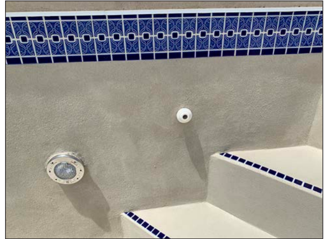
Figure 88: Finished ICF pool steps, plumbing and lights. Ready for the pool season.
