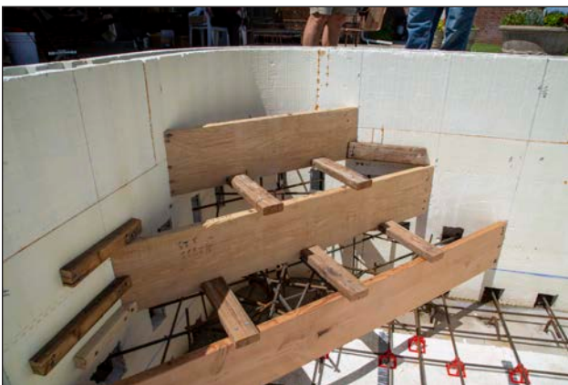
Figure 33: ICF pool steps formed and reinforced. Rebar is tied into the wall at reinforcement at each level.
