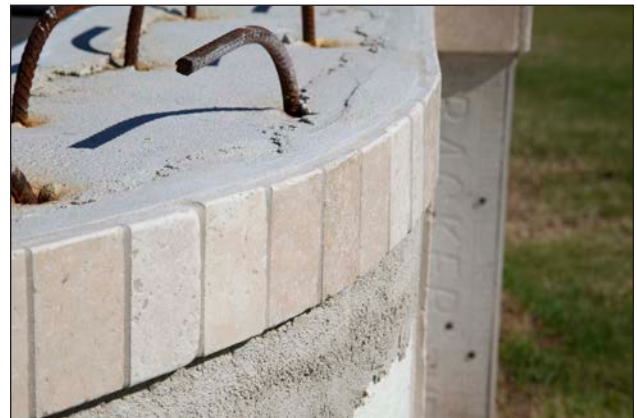
Figure 82: BaseCrete used as a tile bed on pool exterior.
