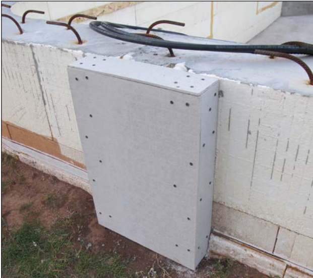
Figure 42: Framed covered with HardieBacker® Cement Board for tile and finish.
