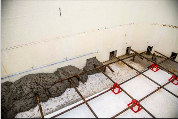
Figure 51: Pouring ICF pool walls.
