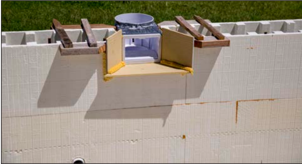
Figure 36: Pool skimmer installed, front face formed and strapped.
