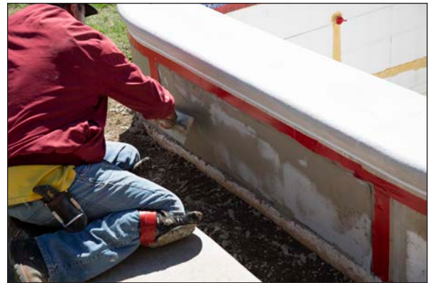
Figure 75: A skim coat is first applied, then the 11oz. mesh embedded and the material is troweled or sprayed to its full thickness and finished.
