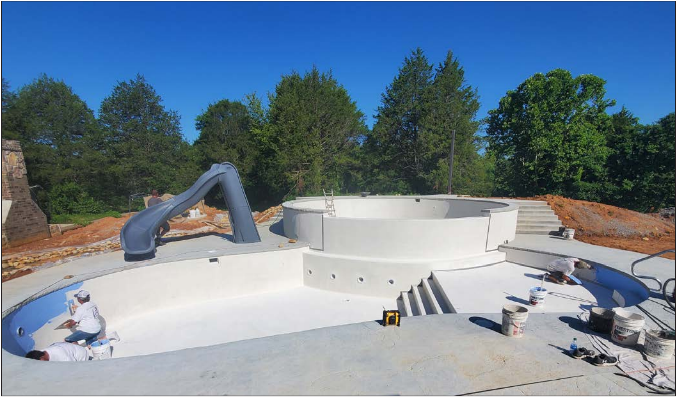
Figure 57: Complex ICF pool finished with BuildCrete Pool Plaster and painted with an epoxy colored paint.
