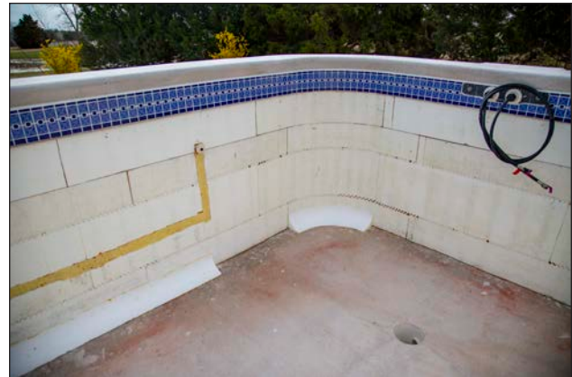
Figure 63: With tile set prepare to install the foam floor to wall cove transition.
