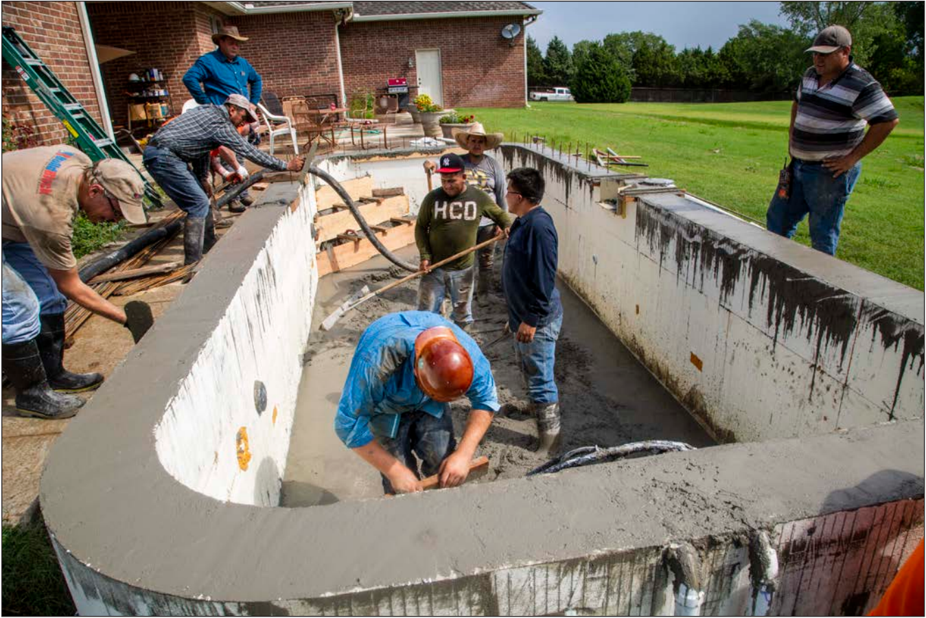
Figure 1: Pouring the ICF walls and floor of a pool.
