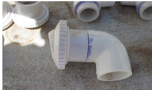
Figure 44: Pool return jets premade to correct length to match with pool finish.
