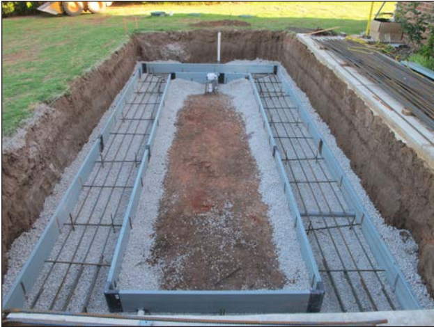
Figure 20: Rebar placed off the ground in the proper place for footing reinforcement.
