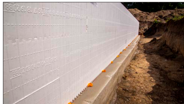
Figure 28: Two courses of ICF wall stacked, shimmed and trimmed, spot glued in place.
