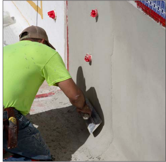
Figure 84: Build up to final thickness and troweled smooth.
