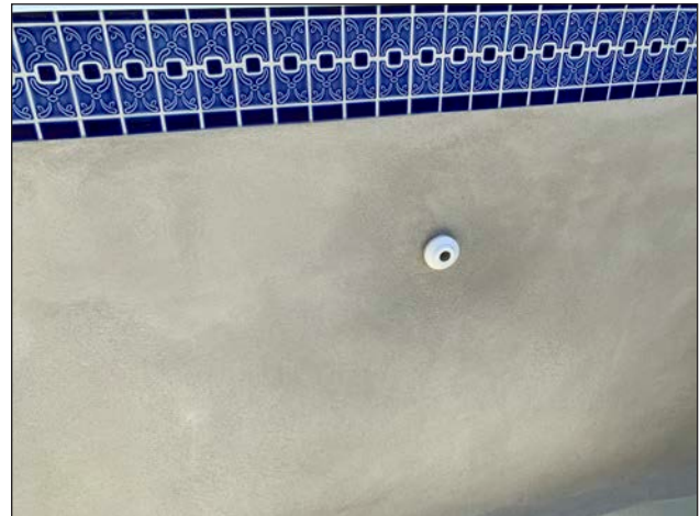
Figure 89: Smooth wall finish.
