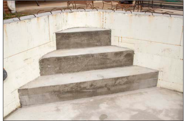
Figure 34: ICF pool steps poured with forms stripped.
