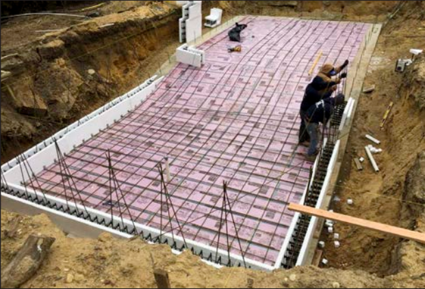
Figure 17: ICF pool with sloped footing.
