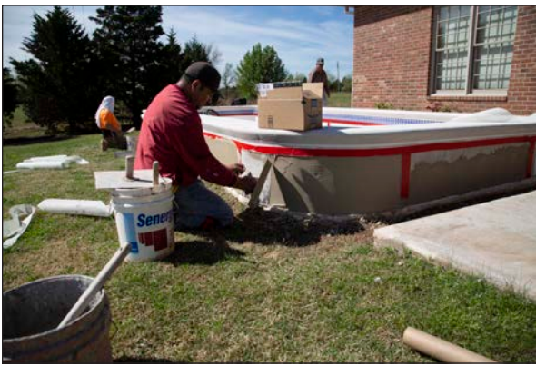
Figure 78: Apply the mesh in sections on curved walls, overlapping as needed. Build up to the desired thickness and finish.
