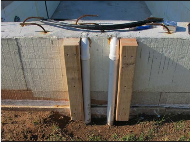
Figure 41: Hydraulic lines for Fastlane Swim in place system installed and framed for HardieBacker® Cement Board for tile and finish.
