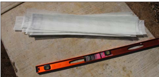
Figure 62: Stage all materials before applying base and setting tile.
