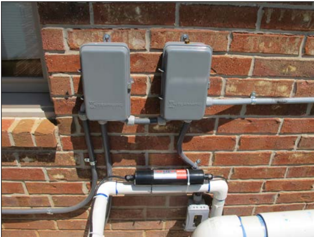
Figure 98: Place all controls so they are easily accessible.
