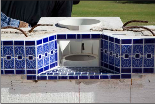
Figure 66: ICF wall prepared with rebar bent and ready to form coping.
