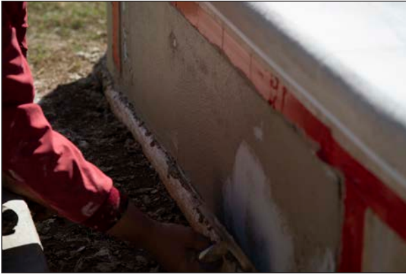
Figure 77: Continue working the material until the full thickness and desired finish is achieved.
