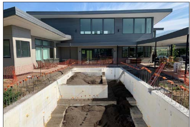
Figure 16: ICF pool with step footings.
