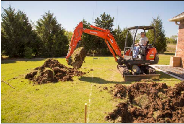
Figure 11: Elevations & finished pool dimensions established.
