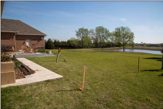
Figure 12: Keep all benchmarks established throughout the pool building process
