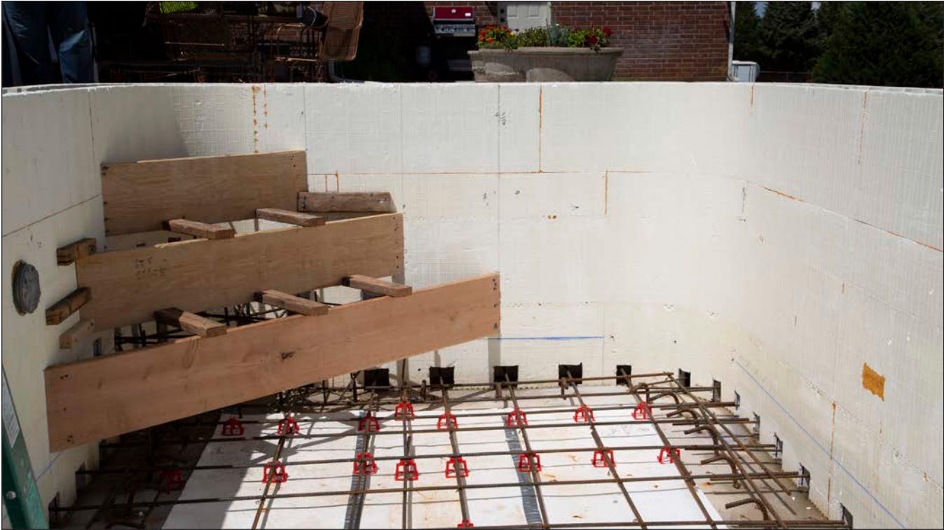
Figure 30: ICF pool steps poured with tile applied.
