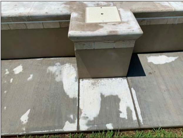
Figure 92: Finished coping and skimmer
