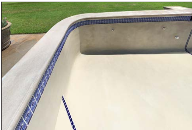
Figure 87: Finished ICF pool with tile ready for the pool season.
