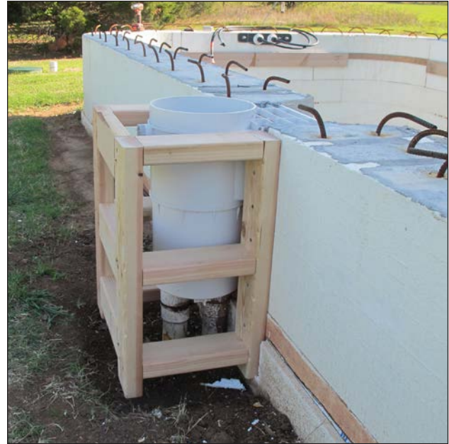
Figure 38: Pool skimmer installed and mounted. Framed and ready for HardieBacker® Cement Board for tile and finish.
