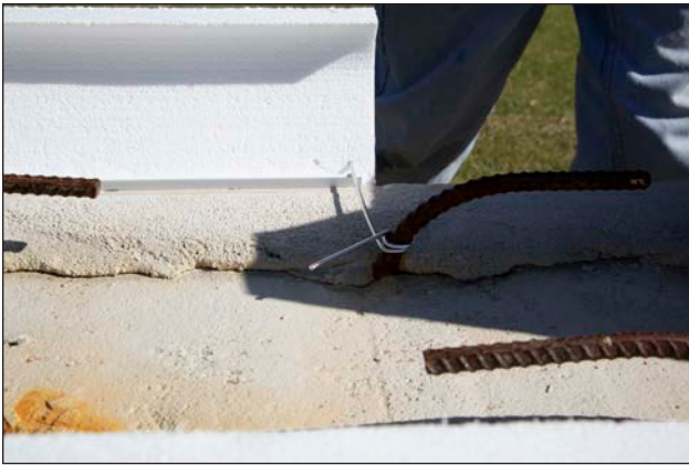
Figure 67: Stegmeier forms are installed and tied to the embedded rebar. After coping is poured the wire breaks away and is left embedded hidden in the coping.
