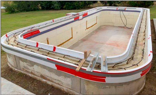
Figure 72: The Stegmeier pool coping forms are installed, wired, reinforced with tape and strapped where needed. Tools are laid out to screen and finish the coping.
