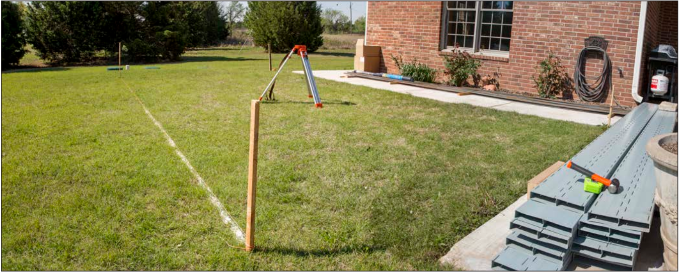
Figure 9: Excavation area marked and benchmark established.
