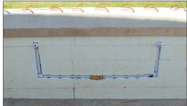
Figure 48: Pool return jets installed, secured in place, and connected to supply line via central coupler passing through sleeve in pool wall.
