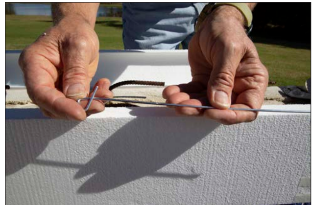
Figure 70: The Stegmeier wire tie is scored to break away after the coping is poured.
