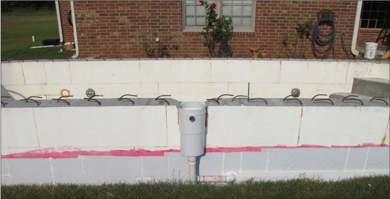
Figure 52: ICF pool with walls poured and waterproofed below grade. This pool uses Form-A-Drain an integrated stay-in-place footing form and perimeter drainage system.
