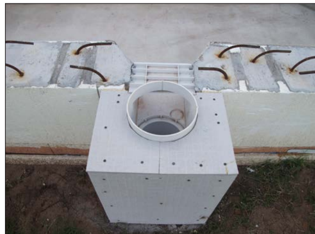
Figure 40: Pool skimmer poured in place and mounted at the correct depth for the coping.
