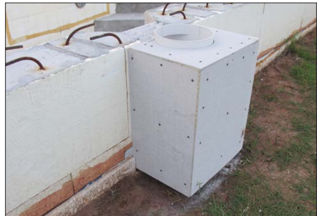
Figure 39: Framed covered with HardieBacker® Cement Board for tile and finish.
