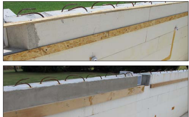
Figure 59: Base installed at top and bottom to ensure level.
