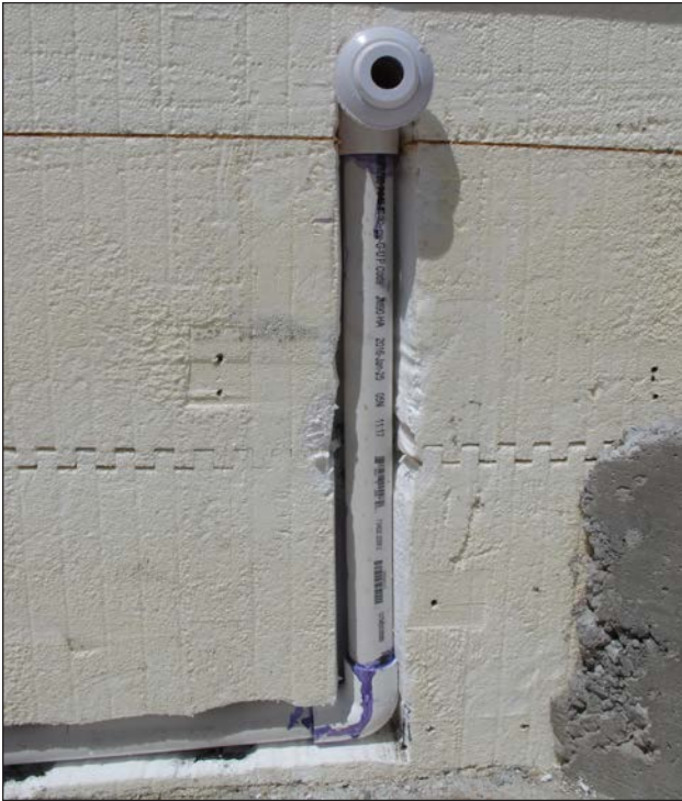
Figure 46: Pool return jet installed.
