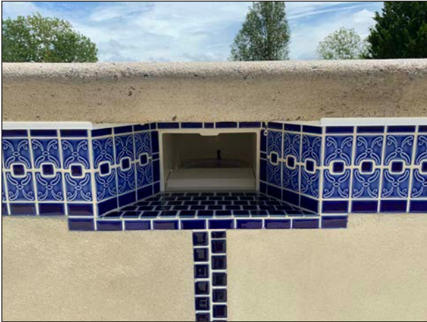
Figure 91: Finished ICF pool skimmer finished with Pool Plaster and tile.
