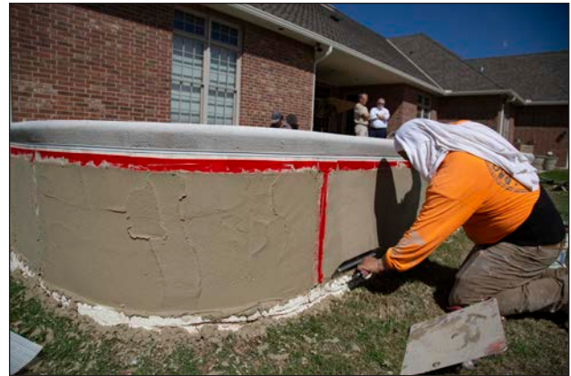
Figure 81: BuildCrete built to final thickness as final smooth finish applied.
