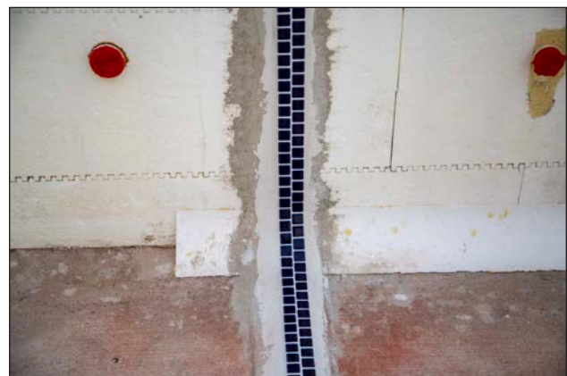
Figure 65: Tile set over floor to wall cove transition.
