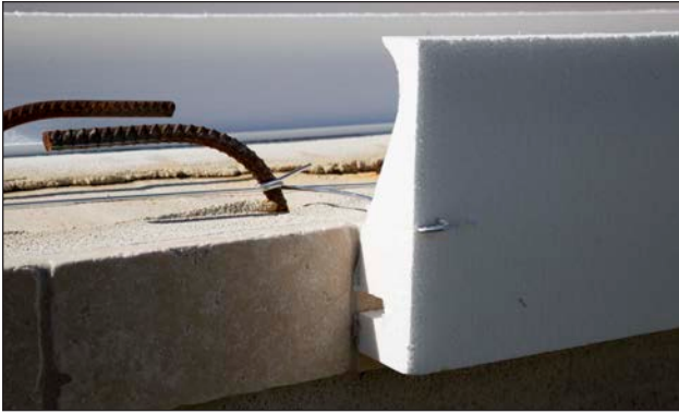
Figure 71: Stegmeier forms are installed and tied to the embedded rebar. After coping is poured the wire breaks away and is left embedded hidden in the coping.
