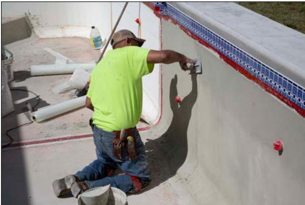
Figure 83: Build up to final thickness and trowel smooth.
