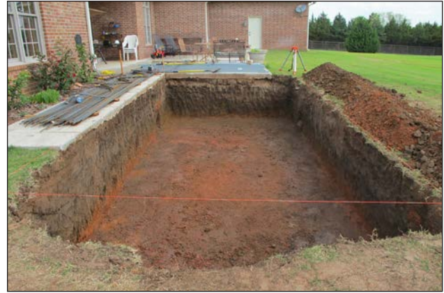
Figure 13: Excavate the hole check finished elevations and depths of the hole
