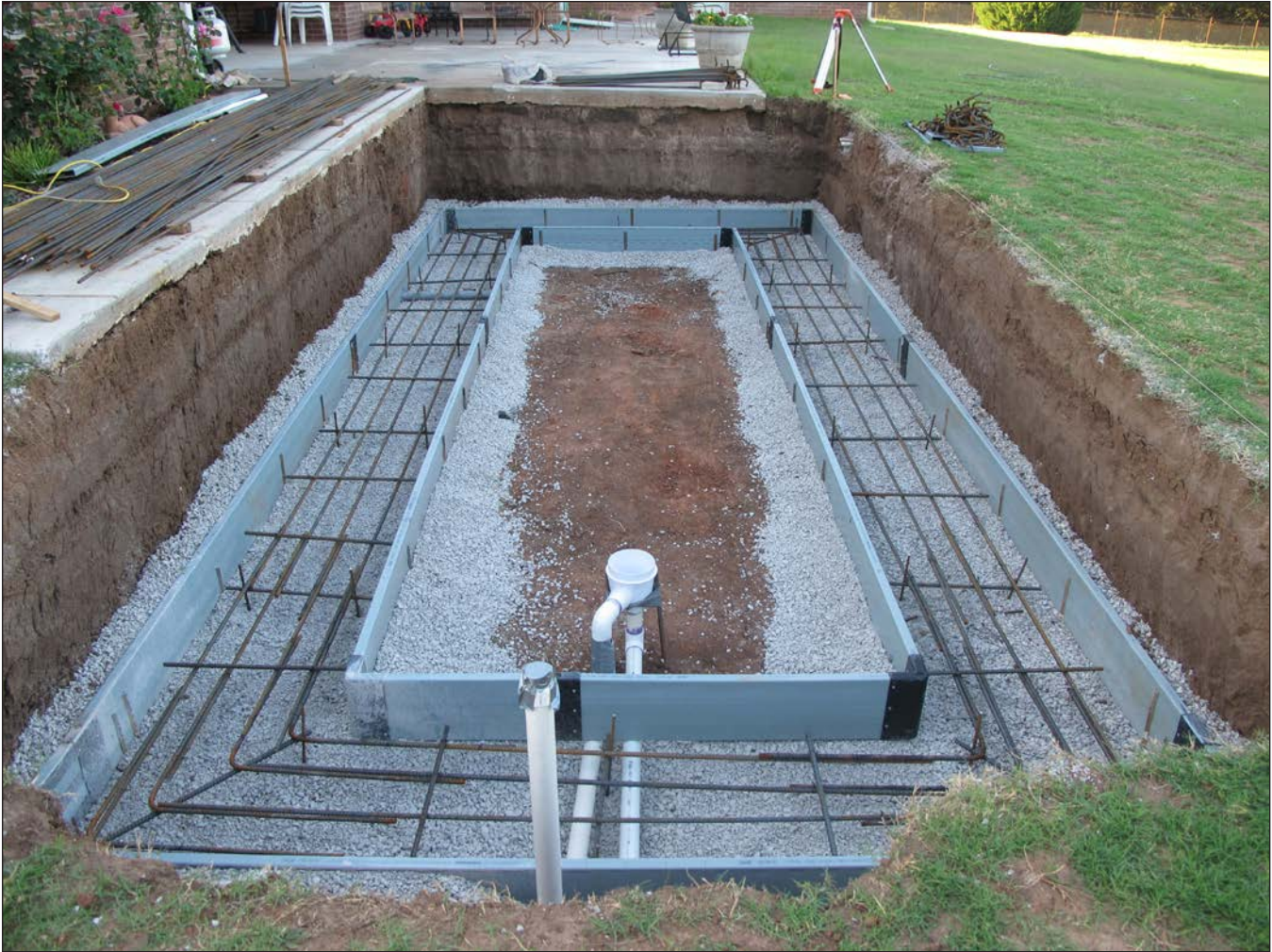
Figure 15: ICF Pool footings formed using Form-A-Drain a stay in place footing forming and foundation drainage system.
