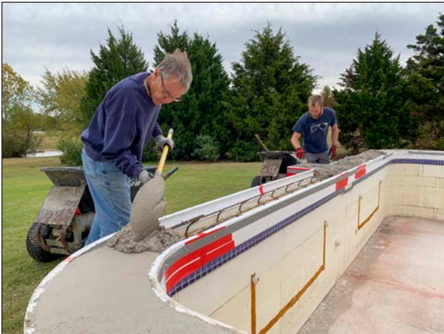
Figure 73: The Stegmeier pool coping is poured using shovels and a concrete hopper. Pour the coping and finish quickly, but fill gently with a high slump concrete and consolidate well for best results.
