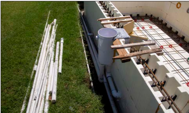
Figure 37: Pool plumbing installed and braced. ICF compatible skimmer installed and strapped.
