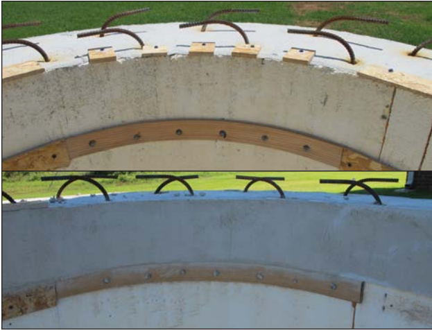
Figure 60: Base installed on top and bottom of curved form to ensure level for tile.
