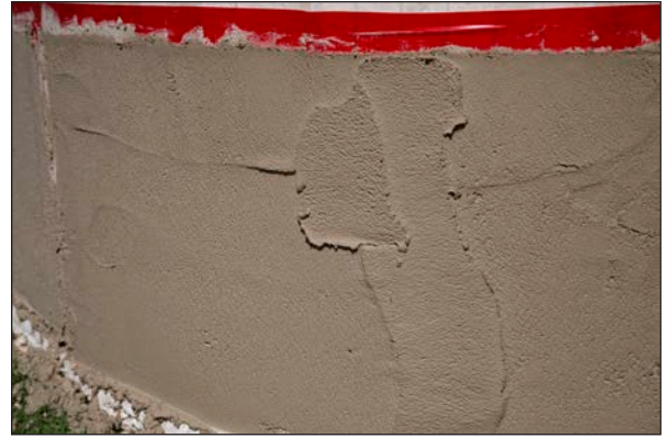
Figure 80: BuildCrete built up to the desired finish before final troweled finish.
