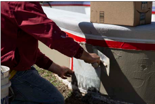
Figure 79: Apply the mesh in sections on curved walls, overlapping as needed. Build up to the desired thickness and finish.
