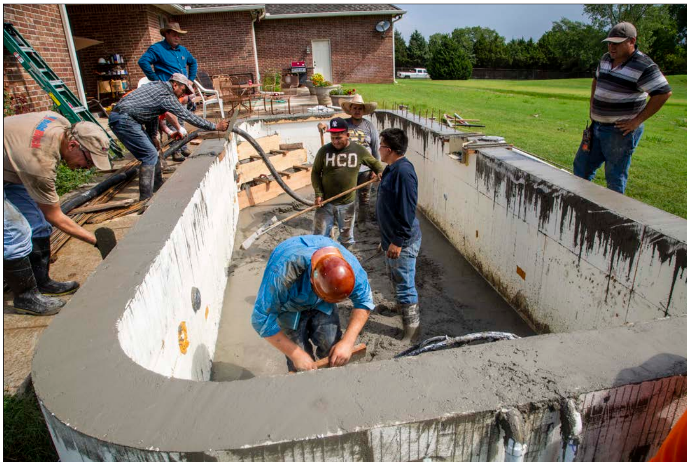
Figure 50: ICF walls and floor being poured using a line pump.
