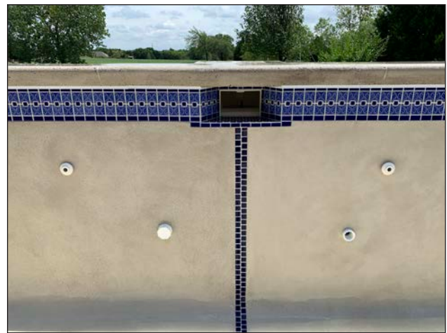
Figure 90: Finished ICF pool skimmer finished with tile.
