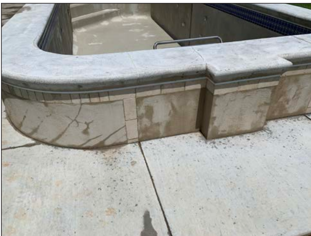
Figure 93: Finished sidewalk, pool coping, and exterior tile.
