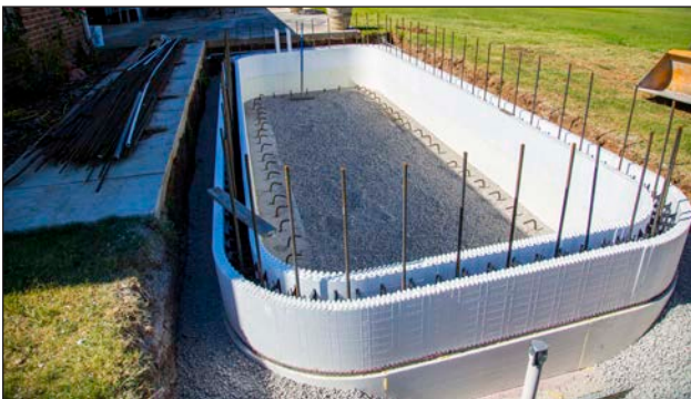
Figure 25: First two courses of ICFs stacked and leveled.
