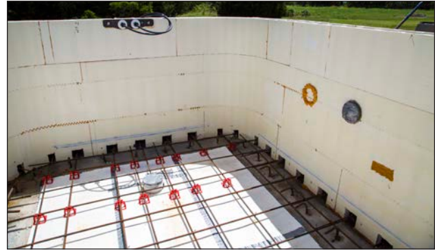
Figure 43: Pool lights sleeves installed and hydraulic lines for Fastlane System. Make sure to protect all sleeves and plumbing from concrete spillage during the pour. If placement errors are made, replace the foam and glue in place. Strap and reinforce as necessary before the pour.
