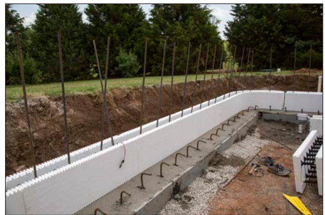
Figure 23: ICF pool foundation poured with vertical rebar dowels and stirrups for the floor.
