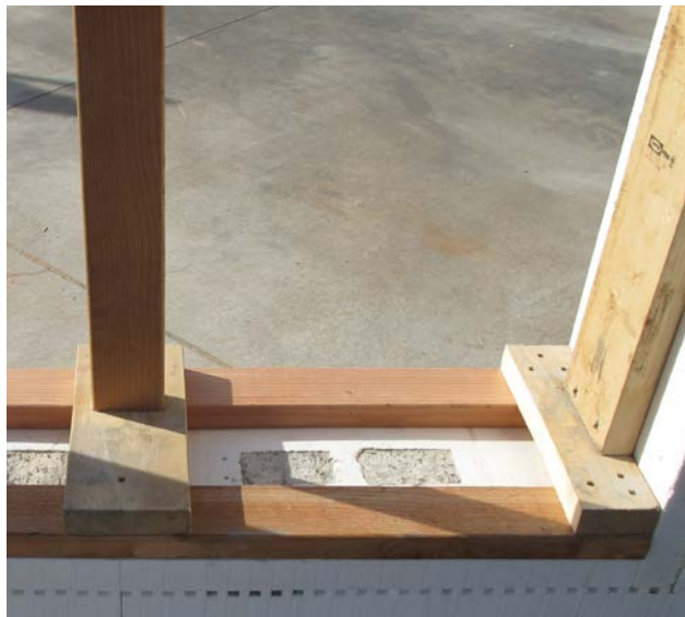
Figure 2.3 Concrete window inspection ports fully filled.
