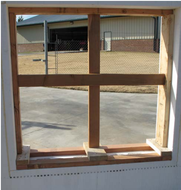
Figure 2.5 Fully cross braced 4040 rough opening.
