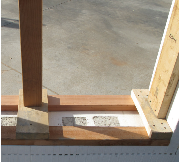
Figure 2.3 Concrete window inspection ports fully filled.
