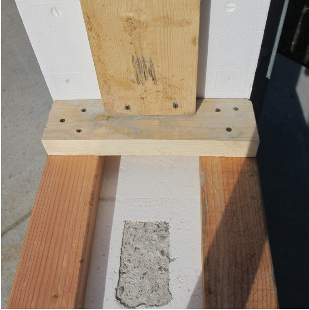
Figure 2.4 Corner bracing properly attached to lateral and longitudinal braces. Side braces attached to buck face.
