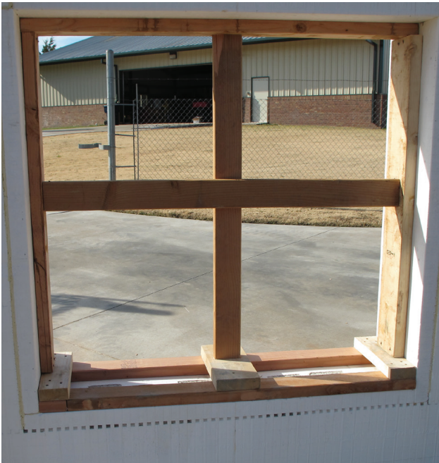
Figure 2.5 Fully cross braced 4040 rough opening.
