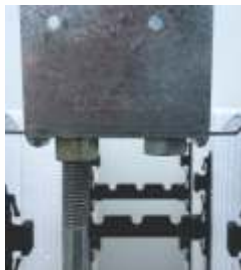
Screw L-Bolt to BHBCON and tighten
