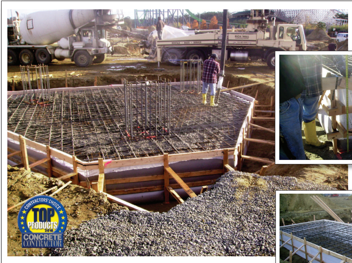
Force Concrete: Six Flags, New Jersey, concrete pads for Green Lantern roller coaster, 42" deep.
