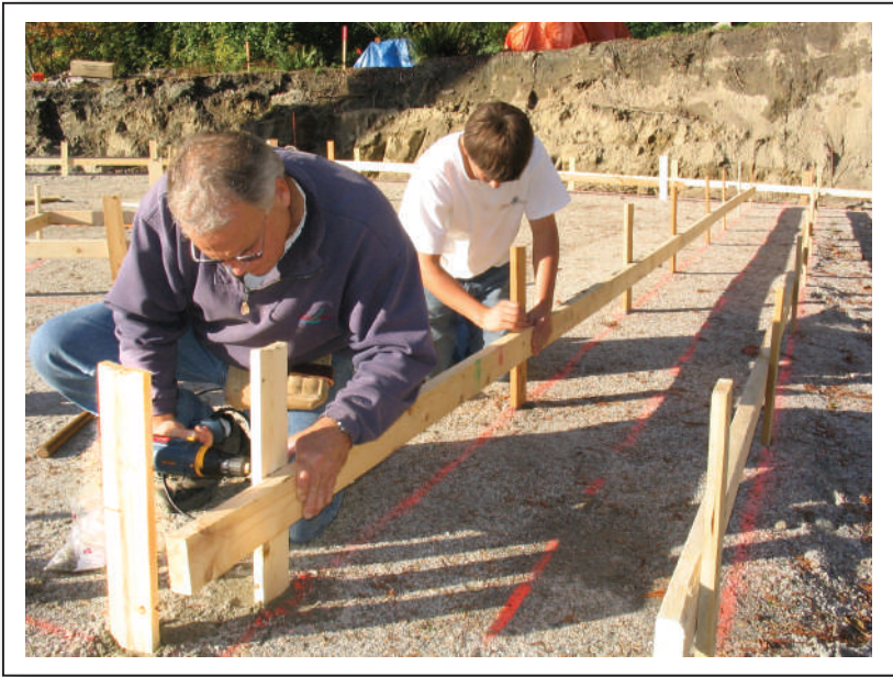
1) Set up screed boards
