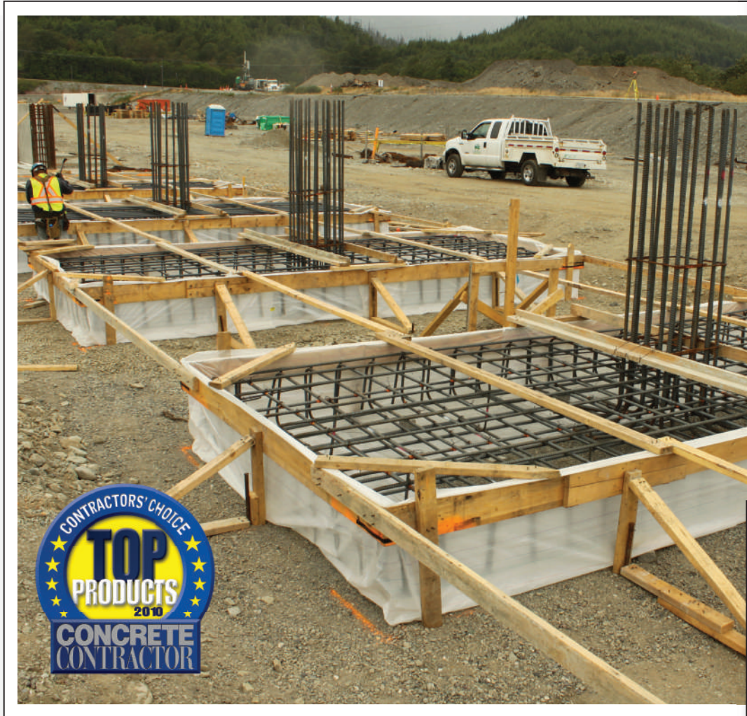
Western Industrial Contractors: Kitimat, BC 145 pads, up to 42" deep.
