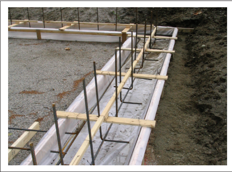
2) Install steel & Fastfoot®
