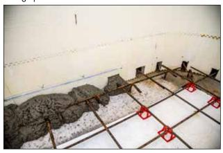
Figure 51: Pouring ICF pool walls.
