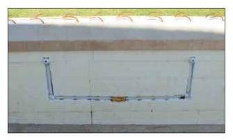
Figure 48: Pool return jets installed, secured in place, and connected to supply line via central coupler passing through sleeve in pool wall.
