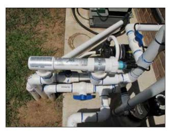
Figure 97: Make sure all plumbing is secured and protected against the environment and is accessible for maintenance as needed.
