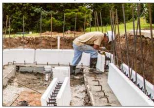
Figure 29: Pool dimensions will not always lay out to block sizes. Use common seams as necessary.
