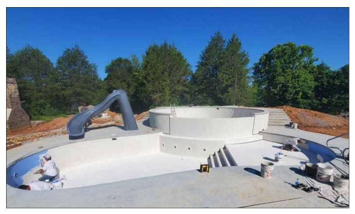
Figure 57: Complex ICF pool finished with BuildCrete Pool Plaster and painted with an epoxy colored paint.
