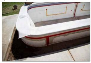
Figure 64: With the cove transition and pool cleaned for finish installation, stage mesh and other materials as needed.
