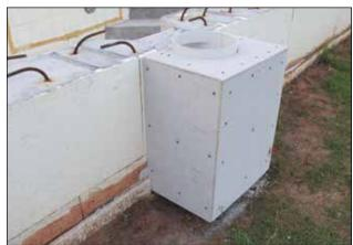
Figure 39: Framed covered with HardieBacker® Cement Board for tile and finish.
