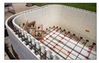
Figure 31: ICF pool floor reinforcement tied into wall reinforcement provides additional strength.
