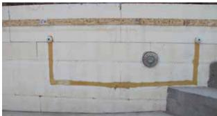
Figure 49: Pool return jets secured in place with foam adhesive and trimmed smooth for pool finish. Electrical light installed and ready for finish installation.
