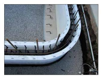
Figure 26: ICF pool wall with vertical and horizontal rebar. Placed either side of center each course a vertical chase is created to hold rebar in place.
