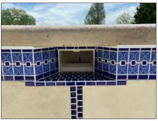
Figure 91: Finished ICF pool skimmer finished with BuildCrete Pool Plaster and tile.
