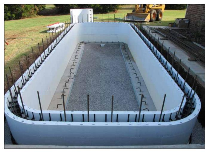
Figure 24: ICF pool walls stacked with reinforcement.
