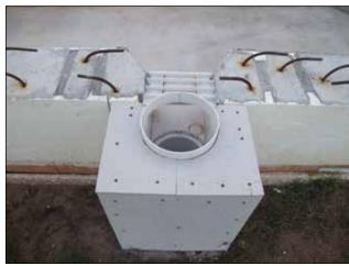
Figure 40: Pool skimmer poured in place and mounted at the correct depth for the coping.
