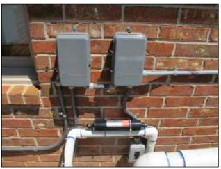
Figure 98: Place all controls so they are easily accessible.
