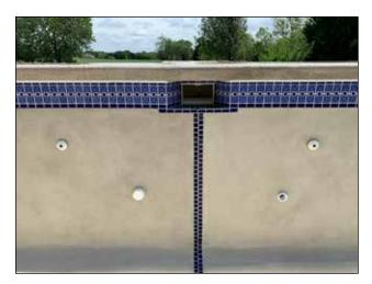
Figure 90: Finished ICF pool skimmer finished with BuildCrete Pool Plaster and tile.
