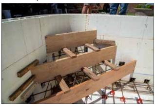
Figure 33: ICF pool steps formed and reinforced. Rebar is tied into the wall at reinforcement at each level.
