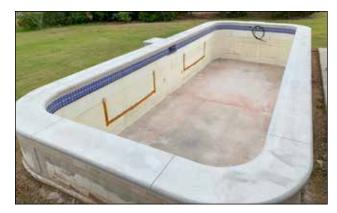
Figure 74: The pool coping is poured and forms stripped. Score with a concrete saw every 24"-36". Fill the seam with pool plaster, caulk, or another material.
