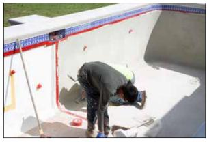
Figure 85: Sectioning the pool for finishes will help ensure a quality finish and prevent overworking the plaster.
