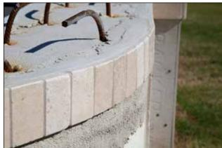
Figure 82: BuildCrete used as a tile bed on pool exterior.
