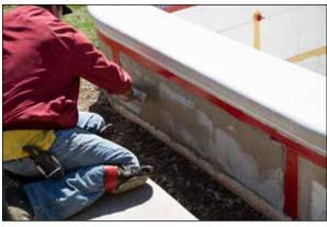
Figure 75: A skim coat is first applied, then the 11oz. mesh embedded and the material is troweled or sprayed to its full thickness and finished.
