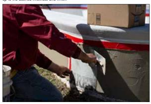
Figure 79: Apply the mesh in sections on curved walls, overlapping as needed. Build up to the desired thickness and finish.
