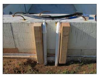
Figure 41: Hydraulic lines for Fastlane Swim in place system installed and framed for HardieBacker® Cement Board for tile and finish.
