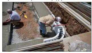
Figure 22: Pouring an ICF pool foundation and screeding the foundation level
