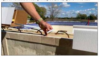
Figure 69: The tile track provides a break between the poured coping and tile to prevent any damage from expansion and contraction.
