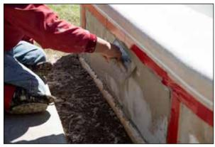
Figure 76: Additional BuildCrete matertial is used to embed the mesh completely and build up to the finshed thickness.
