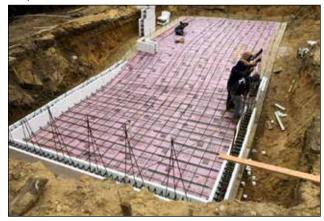
Figure 17: ICF pool with sloped footing.
