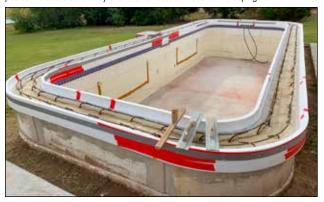
Figure 72: The Stegmeier pool coping forms are installed, wired, reinforced with tape and strapped where needed. Tools are laid out to screen and finish the coping.
