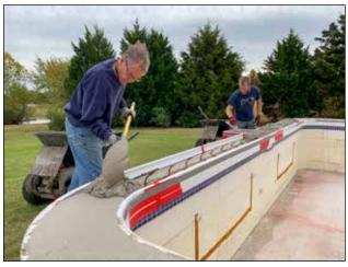
Figure 73: The Stegmeier pool coping is poured using shovels and a concrete hopper. Pour the coping and finish quickly, but fill gently with a high slump concrete and consolidate wel for best results.
