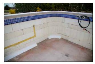
Figure 63: With tile set prepare to insalled the foam floor to wall cove transition
