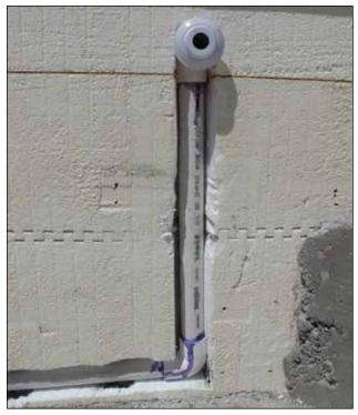
Figure 46: Pool return jet installed.
