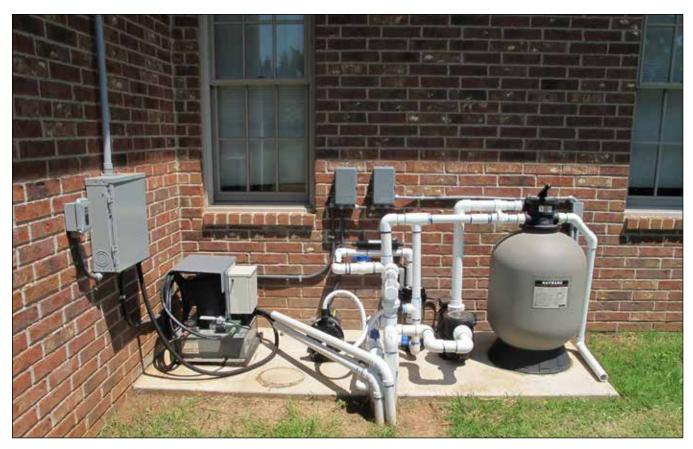
Figure 95: Place pool equipment in a safe area, sheltered from weather with enough space to maintain all equipment and eliminating any hazards.
