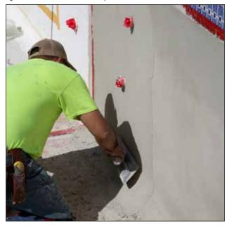
Figure 84: BuildCrete Pool Plaster built up to final thickness and troweled smooth.
